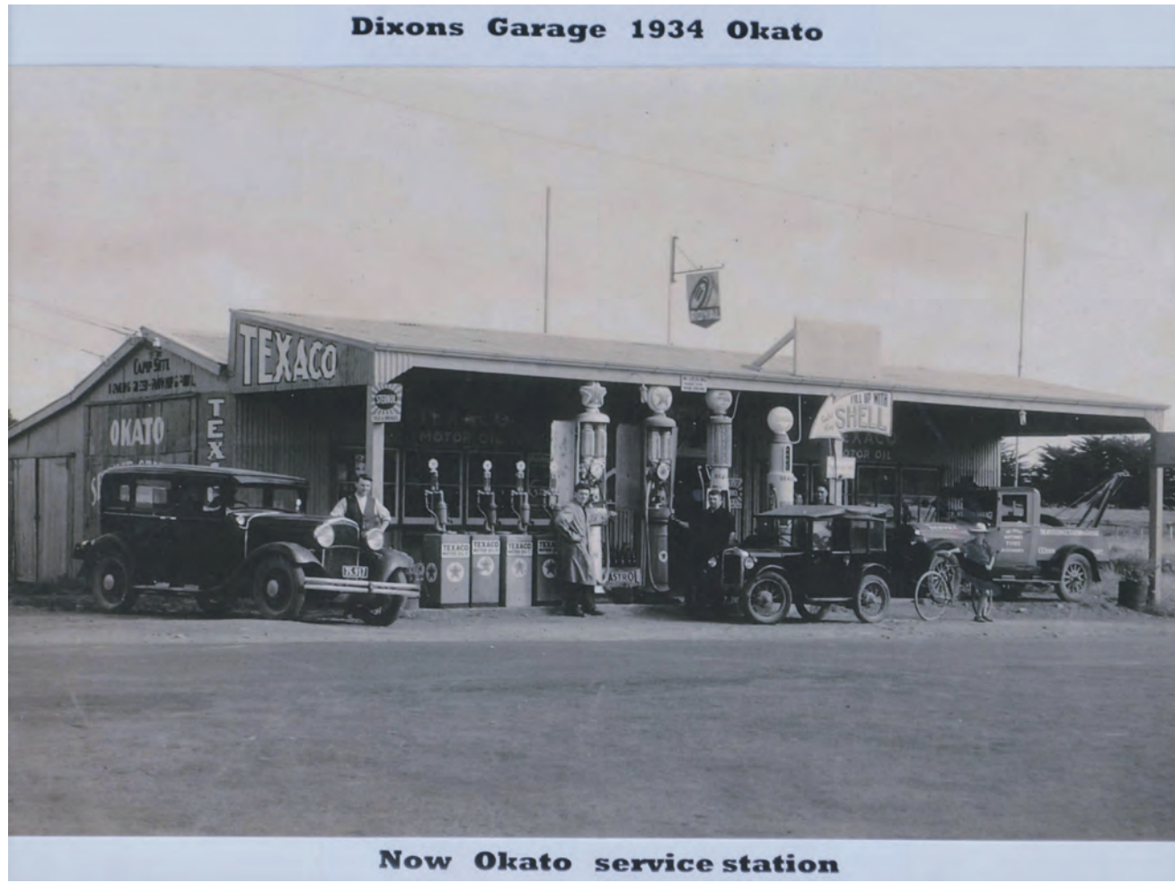
Photo: Lewis Wilson left Trevor and Claude. (Trevor married Miriam Honeyfield). In the 1990’s Kevin Smith owned the garage for a approximately 30 years and was highly skilled in restoring vintage cars similar to the ones in the photograph. He was the last service station owner. He cared for my 1948 Morris Minor.
